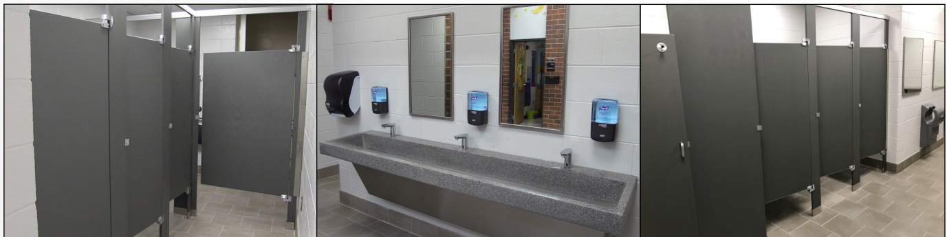
In 2018, voters approved a referendum to complete several projects at Parkside Elementary and Monroe Middle School. At both schools, restrooms were updated to be ADA compliant and improve accessibility for all students, staff, and visitors.
